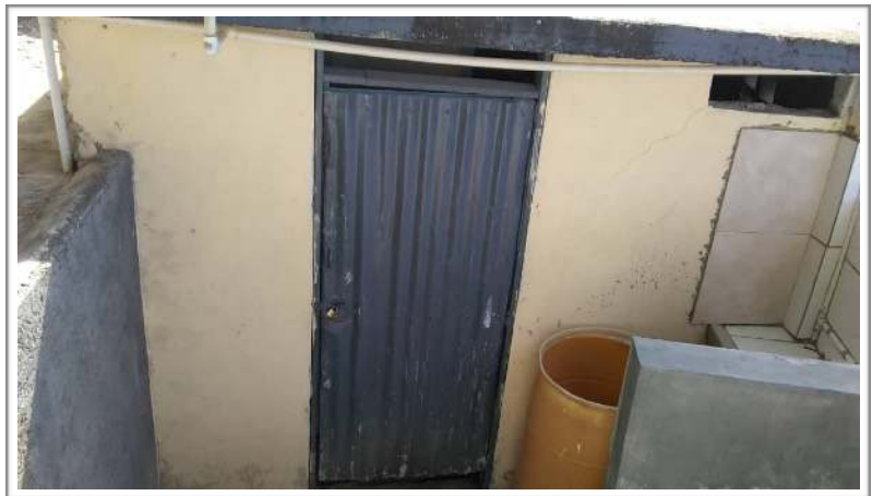
Toilet at St. Joseph Church
