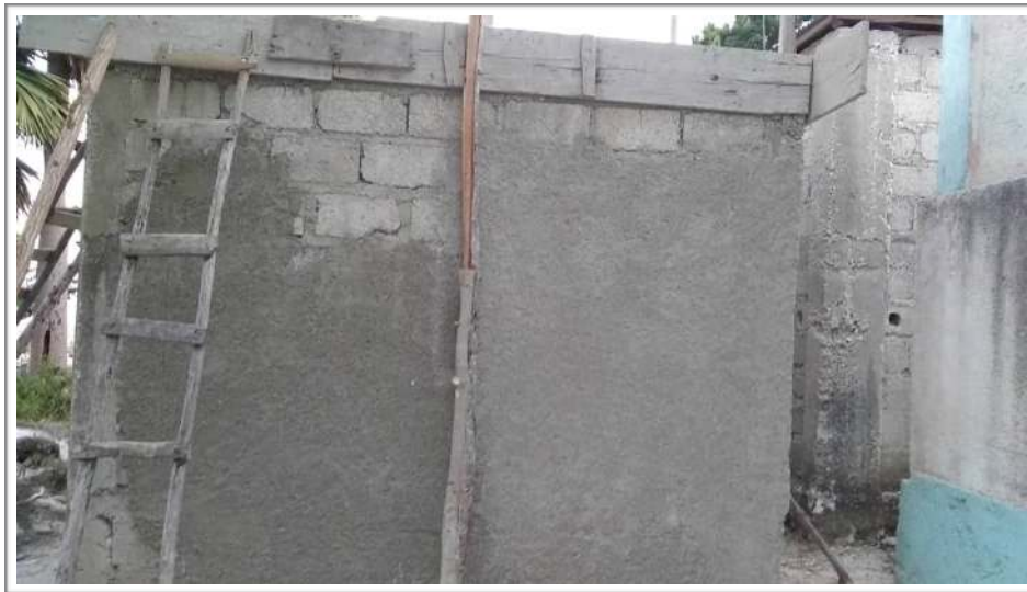
Cistern at Sacred Heart gets a finishing coat of cement.
